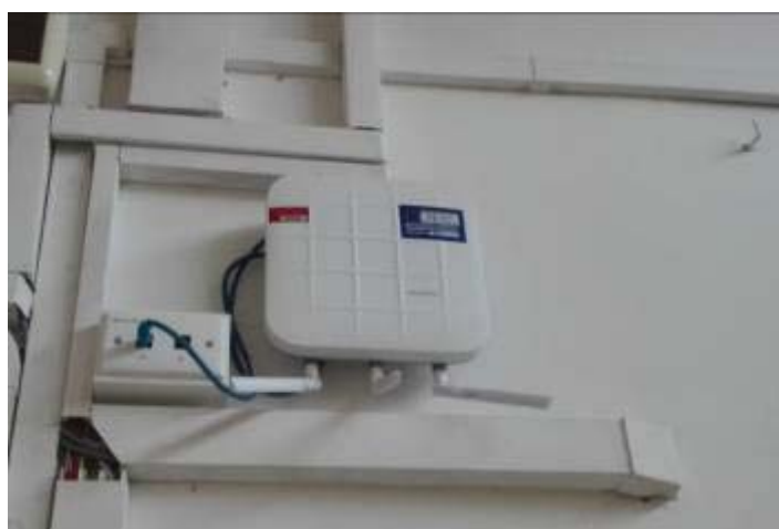
Access Point installati
